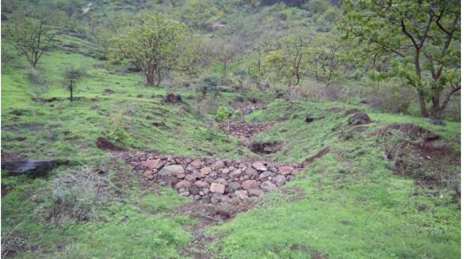
Image of Structures constructed under the Watershed Management Programme , Maharashtra
